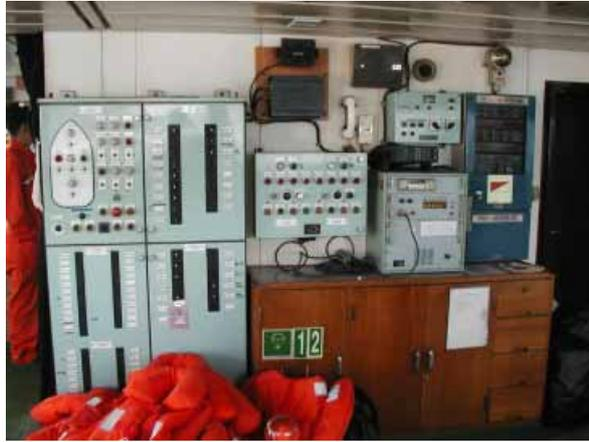
[Fig. 5-4] Various safety panels installed on the wall without ergonomic concept
