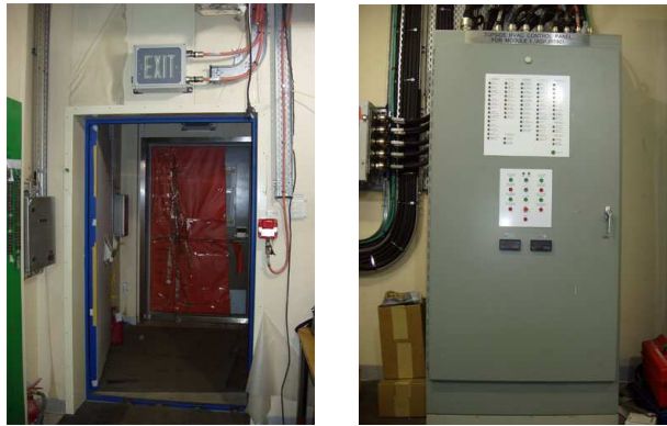
Fig. 4.8 Air lock and HVAC control panel for control module
