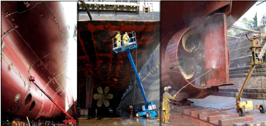
Fig. 1.1 Conventional hull cleaning method
