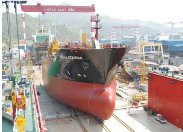
Fig. 2.2 Load Out using Rail
