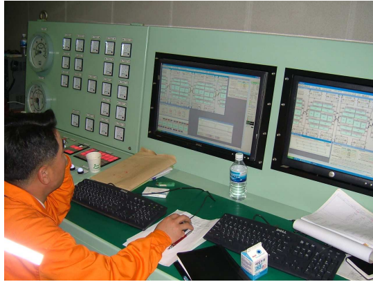
Fig. 2.8 Control Workstation PC in BCR
