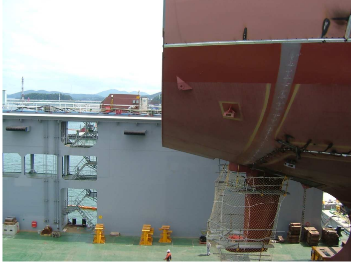
Fig. 3.5 Load Out to Floating Dock
