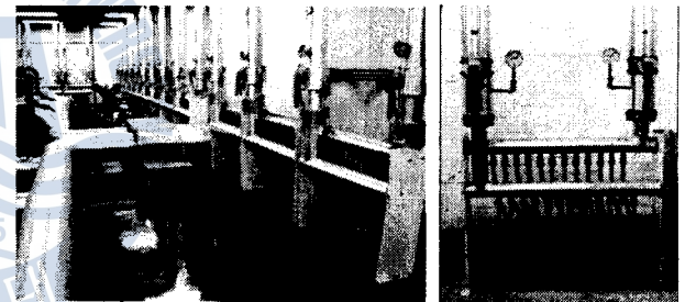
Fig. 3 Header of GHEX pipes
