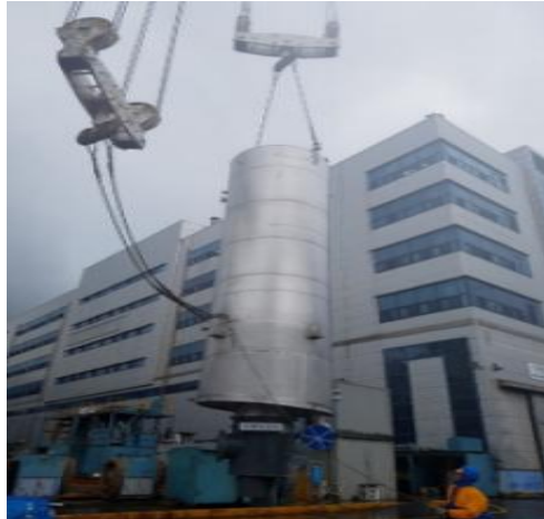
Fig. 3.11 Retrofit of SO x scrubber
