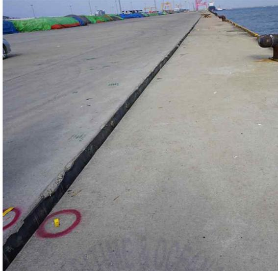
Fig. 4.3 Settlement of caisson (Kim et al., 2019)
