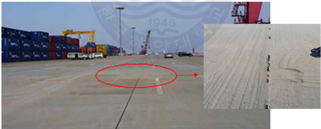
Fig. 4.2 Observed soil boiling (Kim et al., 2019)
