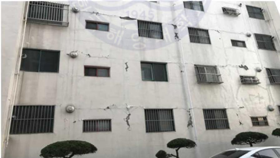
Fig. 1.4 Destruction of external wall due to earthquake in Pohang on November 15, 2017 (Kim and Kim, 2018)
