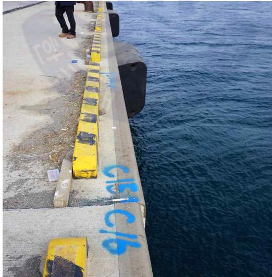
Fig. 4.4 Horizontal displacement of caisson (Kim et al., 2019)
