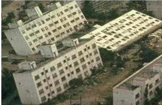
Fig. 1.1 Apartment collapsed due to soil liquefaction in Niigata in 1964
