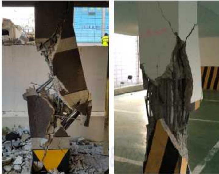
Fig. 1.3 Destruction of pilotis structure due to earthquake in Pohang on November 15, 2017 (Kim et al., 2018)
