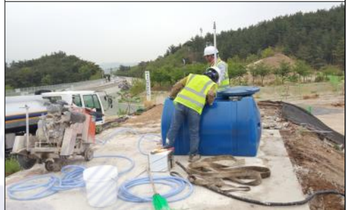
6. Water tank installation
