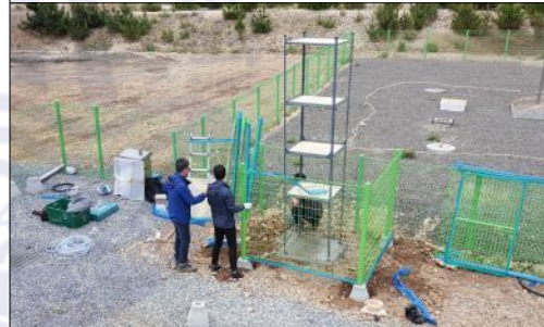
7. Monitoring measure system installation
