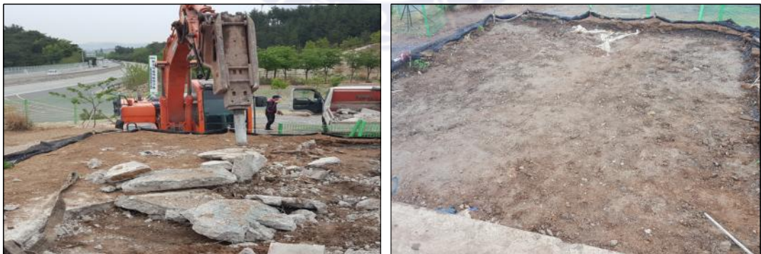
Fig. 4.27 Removing concrete pavement of temporary-stacking section
