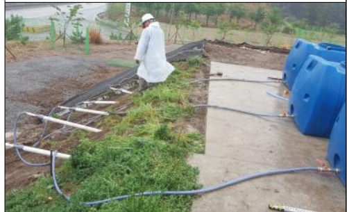
8. Neutralizing & Coating agent injection
