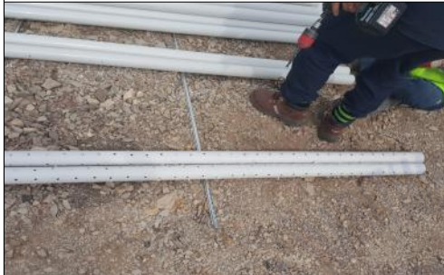
2. Drain pipe perforating
