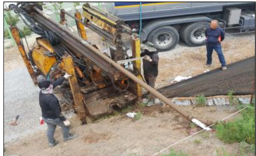
5. Drawing the pipe after insertion
