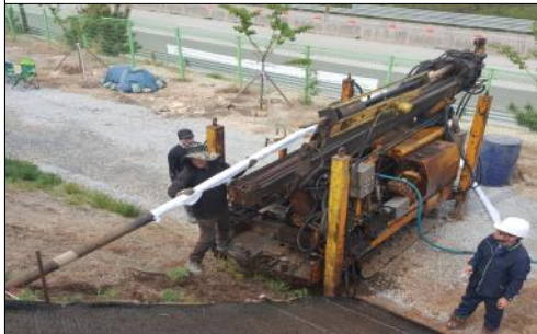
4. Inserting the drain pipe
