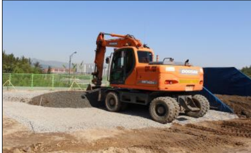
2. Stack the blocking and permeable layer
