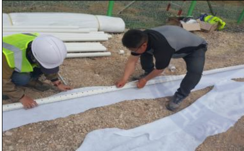
3. Wrap the drain pipe non-woven
