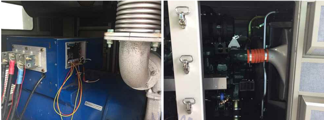
Fig 3.4 Alternator & Variable speed engine
