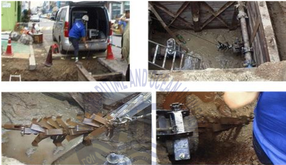
Fig. 1.4 Conventional pipe cleaning method with the scraping tools
